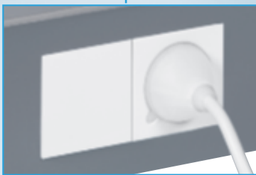
Anti-extraction magnetic socket, for hand-held control device, integrated into the bedhead strip.
