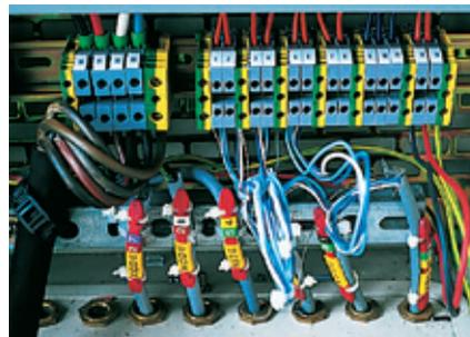
^ Connecting protective conductors by means of Viking green/yellow terminal blocks: the rail is used as collector
