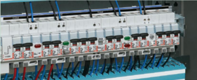
^ Total combination of functions using the Lexic concept. Power, control and signalling are grouped together in wiring areas corresponding to the physical areas of the installation
