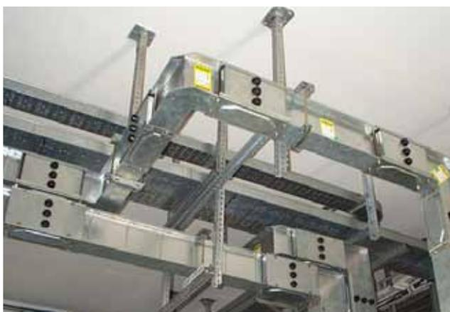
Earth continuity in prefabricated busbar trunking and its connection to the protection circuit are provided by the construction and assembly of the different sections by following the assembly instructions. Other than when requested, there is no specific bar for use as a PE conductor. It is the trunking's steel enclosure which performs this function.
