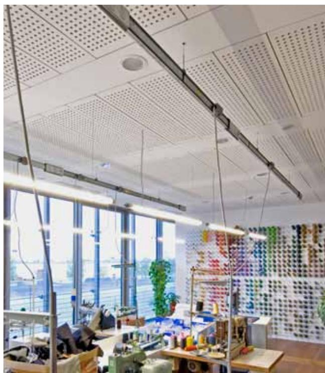
^ Legrand LB low power prefabricated busbar systems in a sewing workshop
