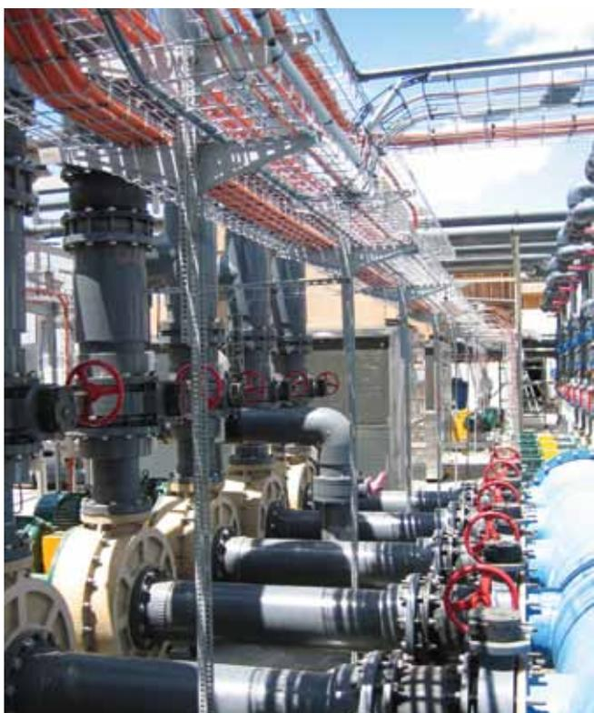
**Wire cable trays used outside in this oil installation supporting cables chosen for their suitability for outside conditions**
