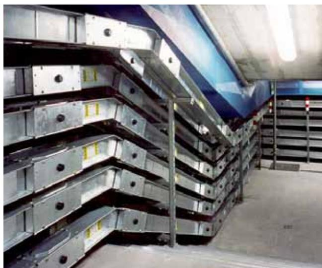
**The prefabricated trunking provides a different response to the requirements in the sense that it includes conductors (busbars) and their insulation (supports) which are protected from external influences by a solid enclosure that defines the protection class.**
