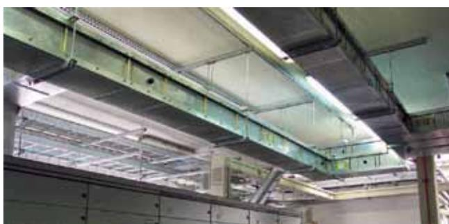
**Prefabricated busbar trunking is constructed to withstand the electrodynamic stresses caused by short circuits within the limits indicated by the manufacturer.**
