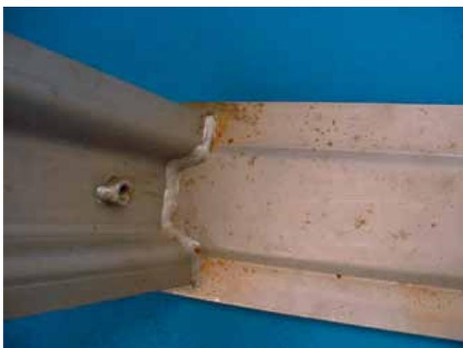
**Traces of corrosion on the stainless steel consoles caused by discharges of iron particles due to grinding or machining assumed to be nearby. A risk that may have unacceptable aesthetic consequences...**
