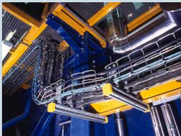
A minimum distance of 100 mm is recommended between the cable trays and the surrounding partitions, walls or ceilings, allowing cleaning devices to pass through easily (source: Nestlé good Hygiene Engineering). Cleaning of cable trays is made easier by installation on consoles in brackets or on hanging fittings. It is more difficult in a sling or when suspended (see fastening methods on page 39).
