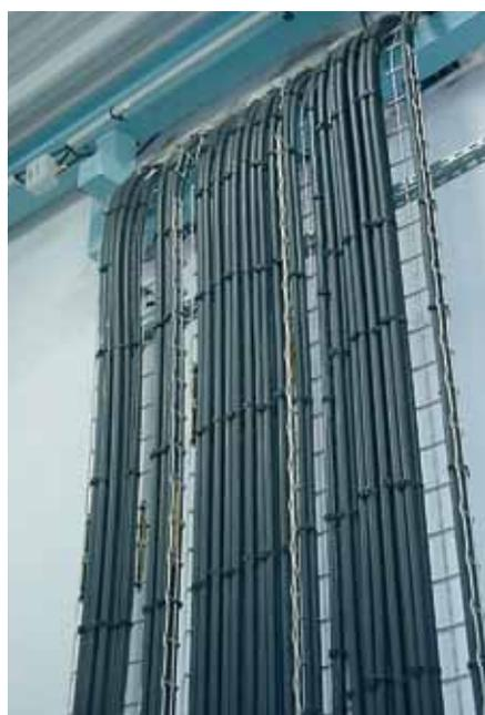
Careful layout of the cables complying with both the grouping rules and the precautions against fire
