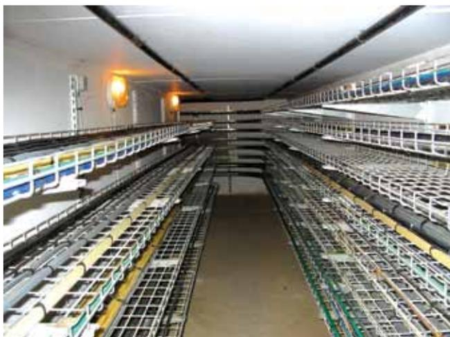
This open structure also ensures very easy cleaning, which makes wire cable tray of great value in the food and chemical industries, purification stations and naval construction.
