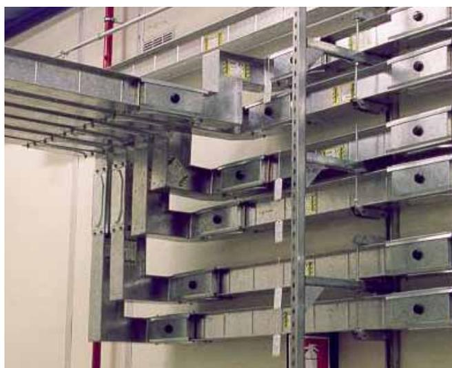
The variety of SCP components allows for any change of direction.
