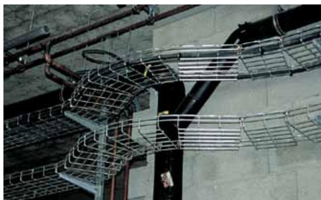
^ The configuration of the site, obstructions, the co-existence of different networks sometimes lead to complex routing
