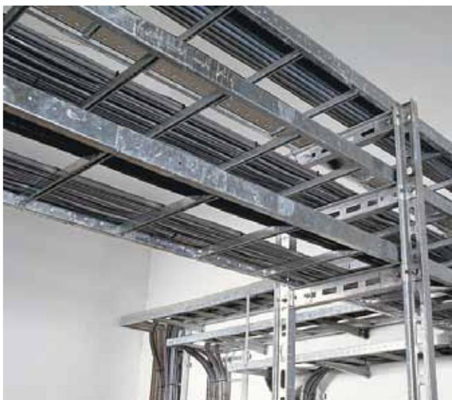
This is the "heavyweight" version of the wire cable tray. The ladder constitutes a support which is suitable for power cables and bundles of a greater weight or size. Its rigidity makes it most suitable for simple (backbone) routes. It is used as a distribution support for all types of cables in protected premises (e.g. technical areas, tunnels). Yet here again, it is the properties of the conductors and cables which determine the resistance to external influences.
