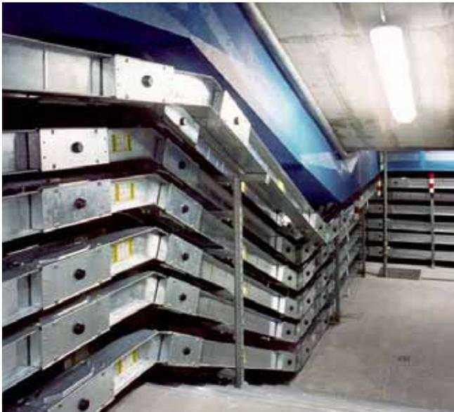
The compact dimensions of SCP trunking allow it to be installed, even in confined spaces.
