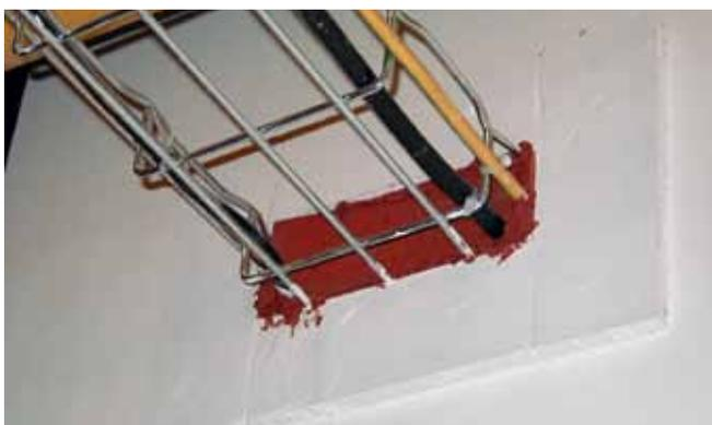
**Filling of a fire barrier partition feedthrough with plaster and intumescent paste**
