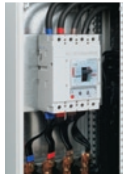
< External cable sleeves are extendable: DPX or DPX-IS 250 and 630
